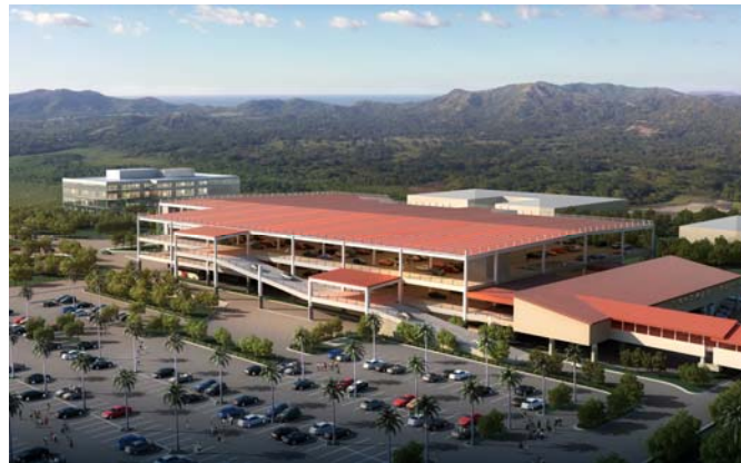
View of RITC, Customer Service Building looking southeast
