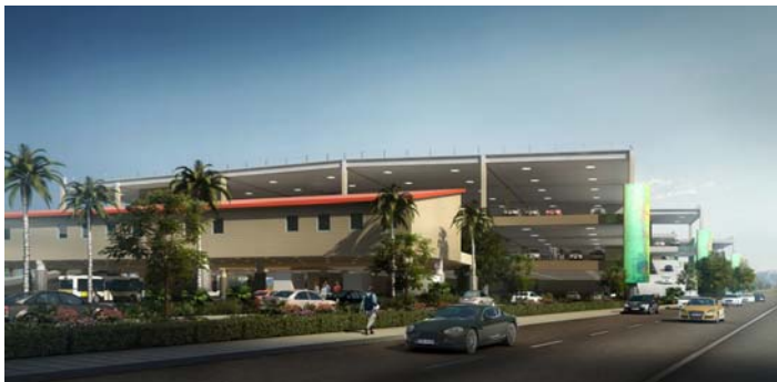
View of Customer Service Building and Consolidated Rental Car Facility looking east from Empire Avenue
